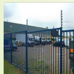
SECURITY FENCE BARRIER SYSTEM
